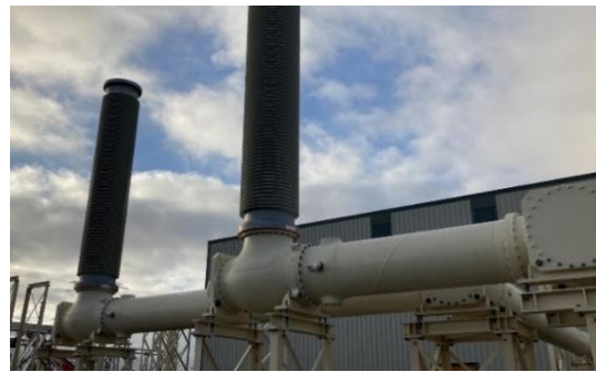
Figure 8 – First installation of a 420 kV clean air GIB – OHL feeder bay
