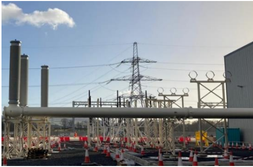
Figure 8 – First installation of a 420 kV clean air GIB – OHL feeder bay
