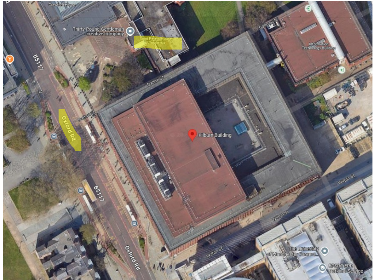
Aerial photo of Kilburn Building location
