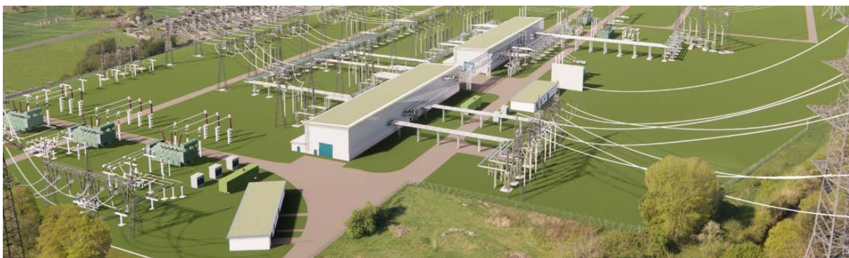
Figure 2. Updated design of the GIS with NOG-based GIBs
