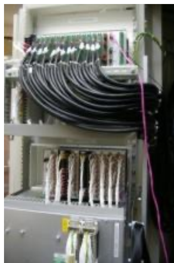
A typical P&C panel (Conventional substation)
