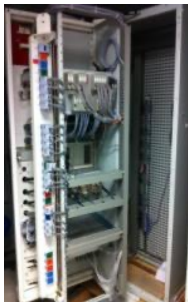
A typical P&C panel (Conventional substation)
