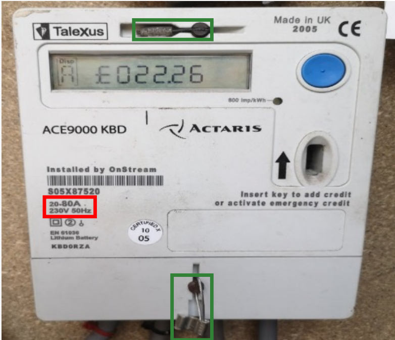
Labelled Image of a Meter
