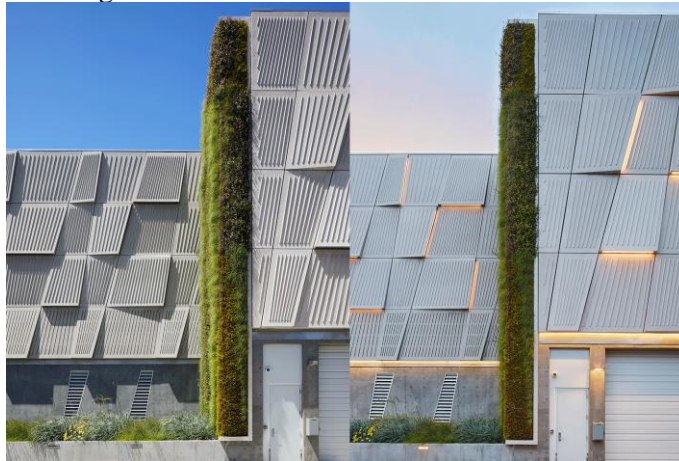
Figure 1: PG&E Larkin Substation outer view during day & night
