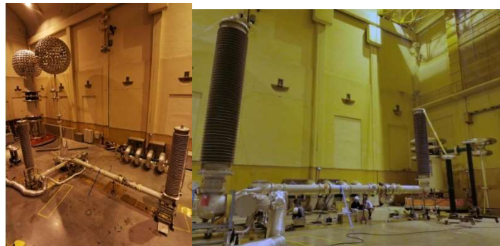
Figure 6 - Bus charging test in laboratory performed on both gases.
