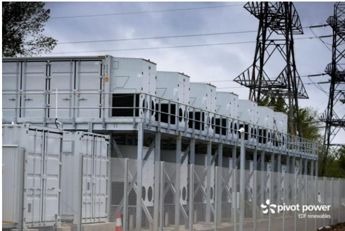
Pivot Power's 50MW BESS in Oxford, UK, 1 st tertiary connection to grid Available at: https://www.edf-re.uk/news-and-views/pivot-power-wartsila-and-habitat-energy-activate-50mw-transmission-connected-battery-in-cowley-oxfordshire/
