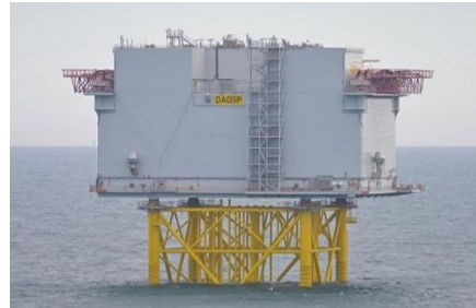
Figure 2: Dogger Bank topside. Credit: SSE [2]
