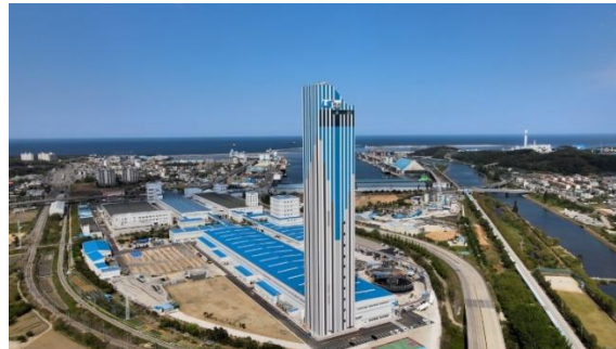
Figure 5: LS Cable & System HVDC cable factory in Donghae, Korea. Credit: LS Cable & System [6]
