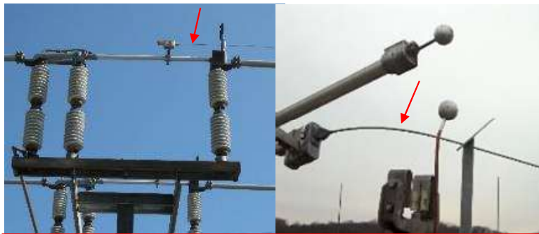
High Velocity Interrupter or Quick Break Device (approx. 15 to 20 A) Note: not used to break load
